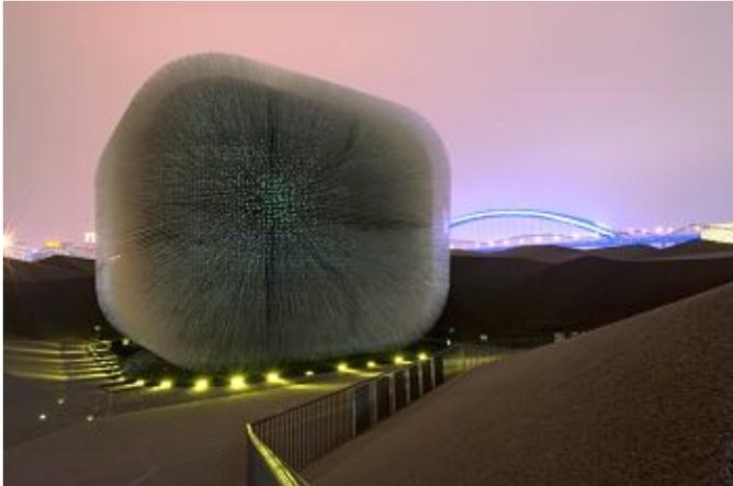
Unofficially called the "dandelion" for its puff-ball structure, the Seed Cathedral portion of the UK pavilion consisted of 60,000 transparent rods bristling from a timber core.
